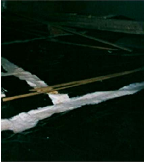
Sealed and Overlapped Seams
