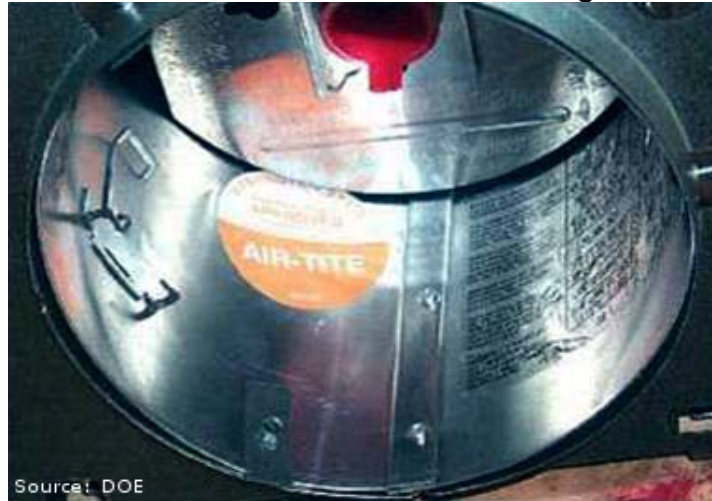
CORRECT: IC-Rated and Air-Tight
