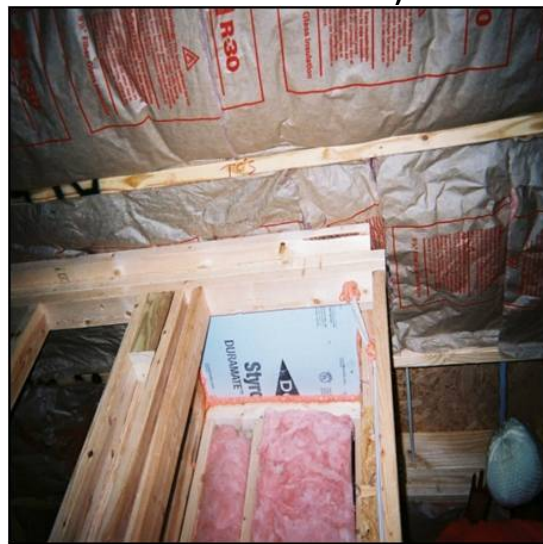
CORRECT: Well-sealed Chase (Prior to Duct Installation)
