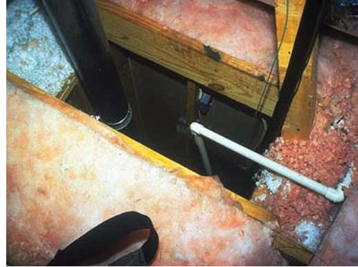
CORRECT: Well-sealed Chase (Prior to Duct Installation)
