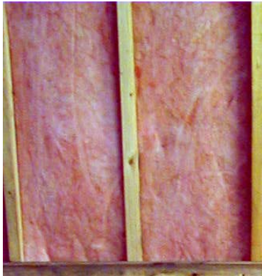
CORRECT: Batt in Wood-framed Cavity
