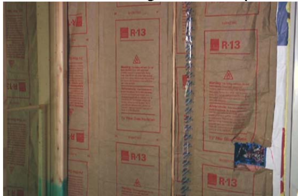
CORRECT: Full Coverage and No Compression
