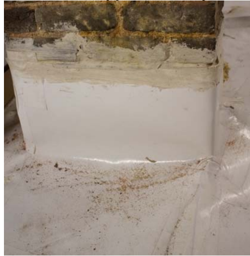
Sealed and Applied 6 in. up Wall
