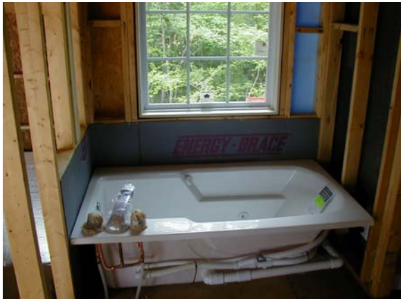
CORRECT: Air Barrier Behind Tub
