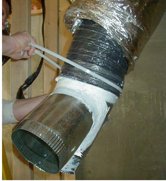
CORRECT: Mastic-sealed Joints
