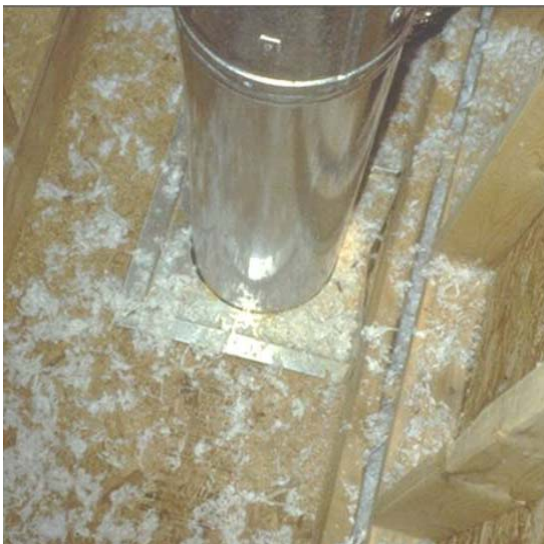
CORRECT: Well-capped Chase
