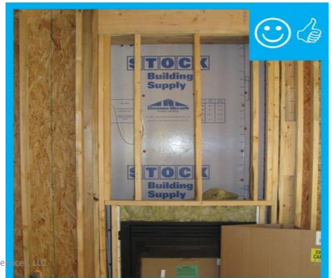
Rigid air barrier over insulation behind fireplace
