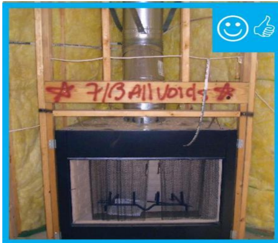
Insulation behind fireplace
