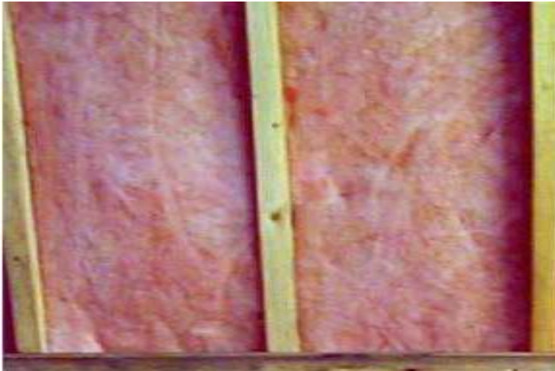
CORRECT: Batt in Wood-framed Cavity
