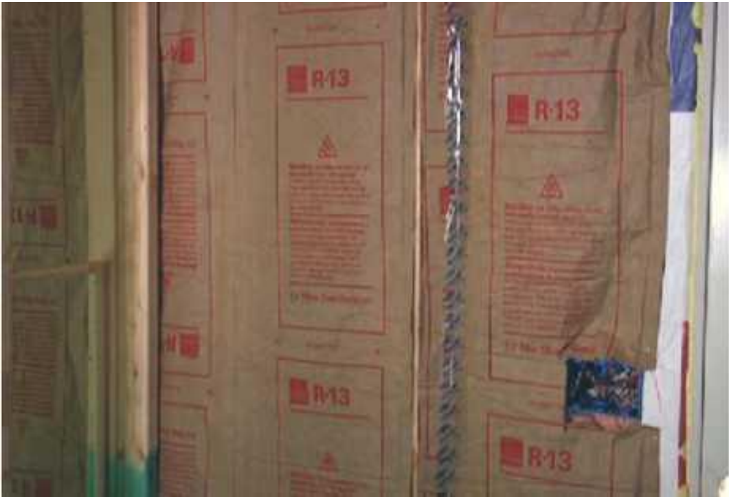
CORRECT: Full Coverage and No Compression
