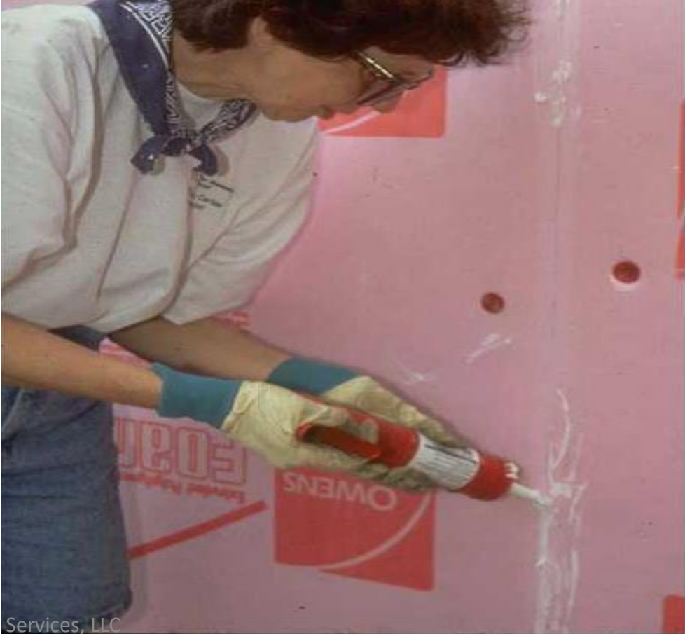
CORRECT: Sealing Exterior Sheathing
